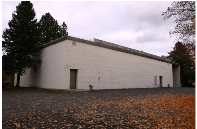
Southwest corner, looking northeast
