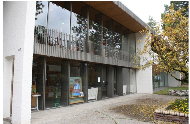
North facade, looking west
