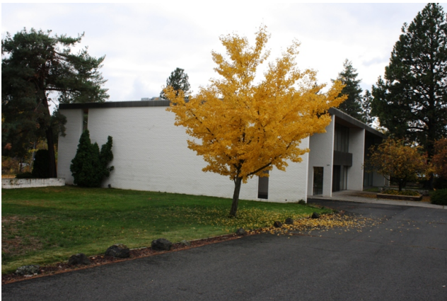
Northeast corner, looking west
