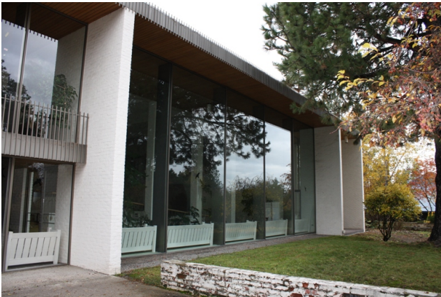
North facade, looking northwest
