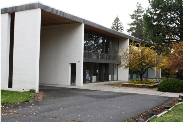
North facade, looking southwest
