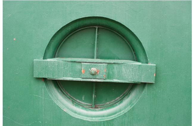
View of hatch at base of reservoir
