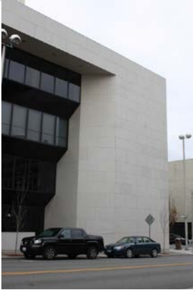
East facade, north side, looking northwest
