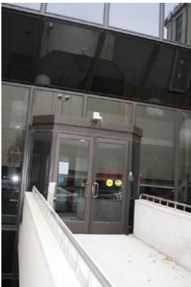
Entry vestibule on north facade
