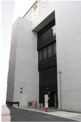
South facade, looking northwest
