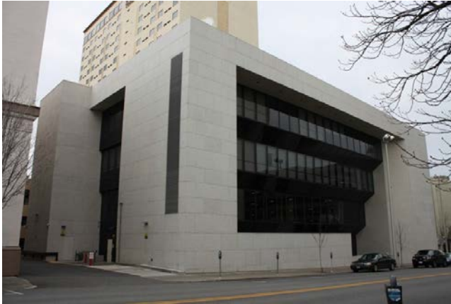
South and east facades, looking northwest
