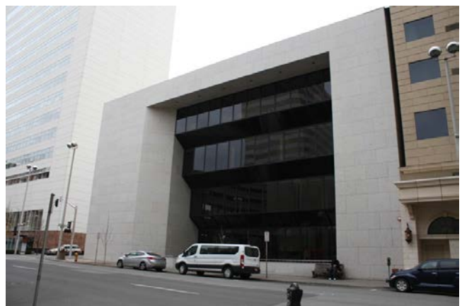
North facade, looking southeast
