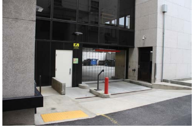
Entry to parking garage, south facade
