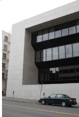
East facade, south side, looking west
