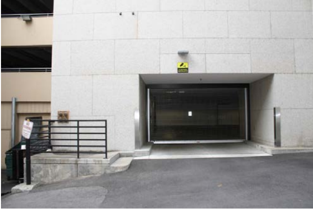
Exit from parking garage, looking north
