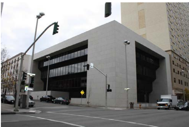
North and east facades, looking southwest
