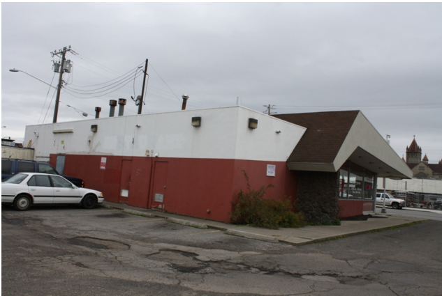
North and west facades, looking northwest
