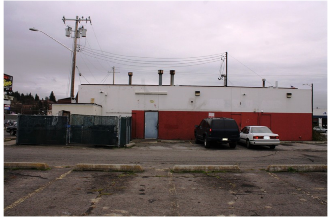
North (rear) facade, looking south
