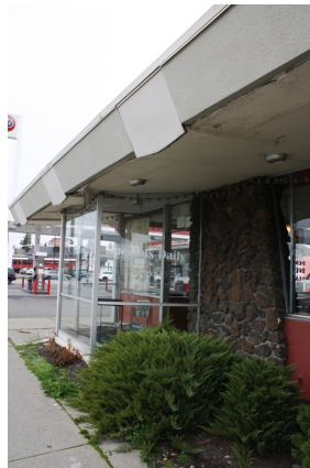
Entry on south facade, looking west
