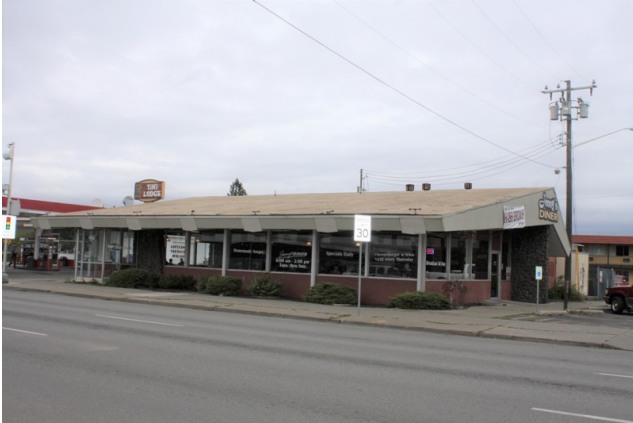
South and east facades, looking northwest
