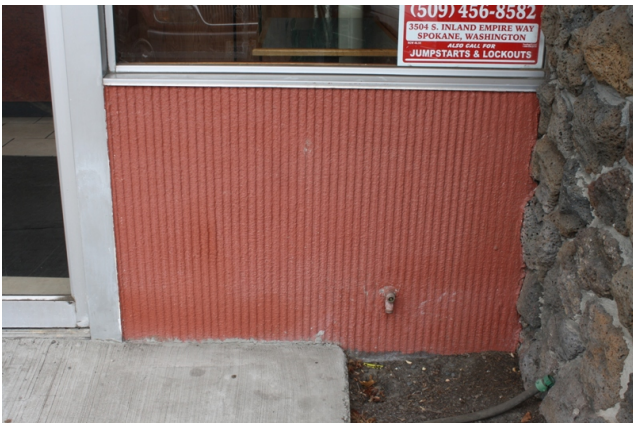
Material detail below window sills
