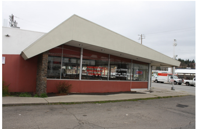
West facade, detail of roof, looking east
