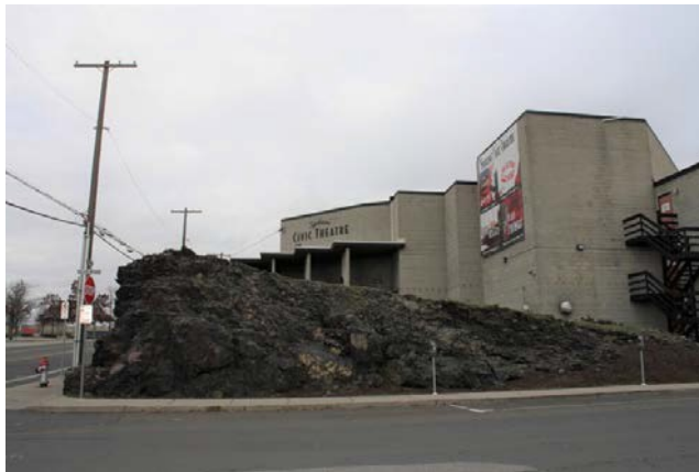
Southwest corner, looking north
