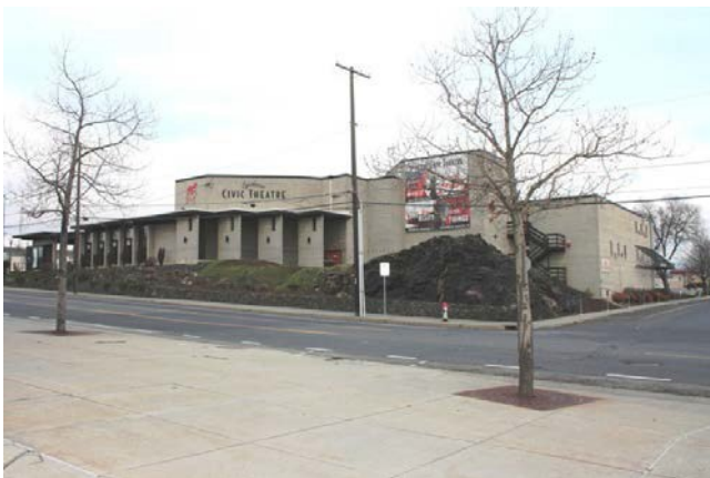
Southwest corner looking northeast
