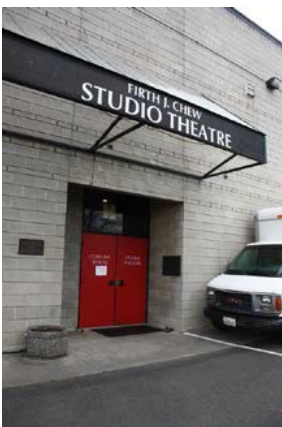
East facade, detail
