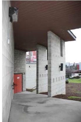
South stair, looking south
