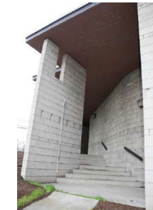
South stair, detail
