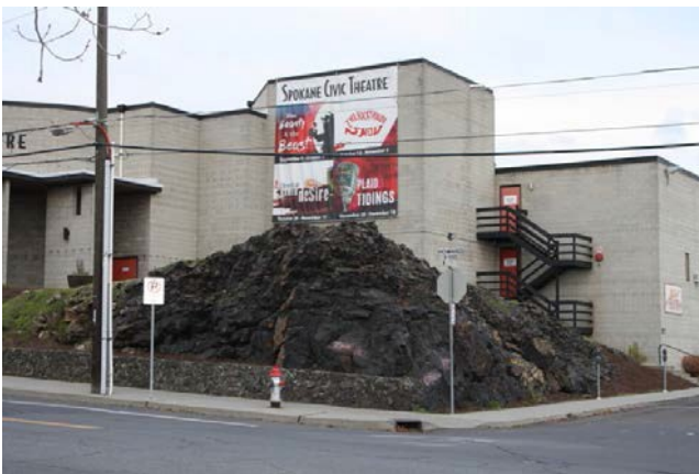
Southwest corner, detail
