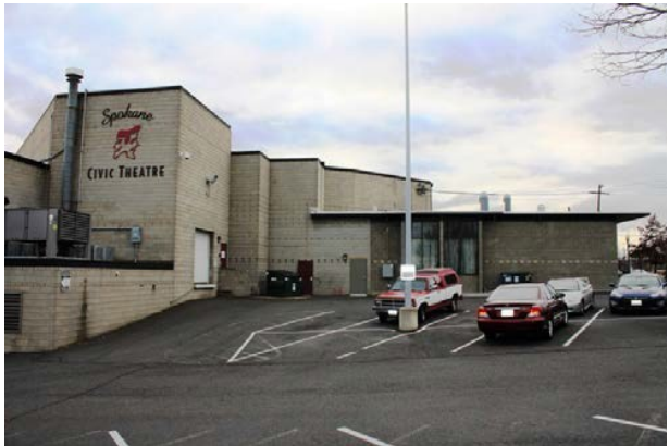
East rear facade, north side, looking west
