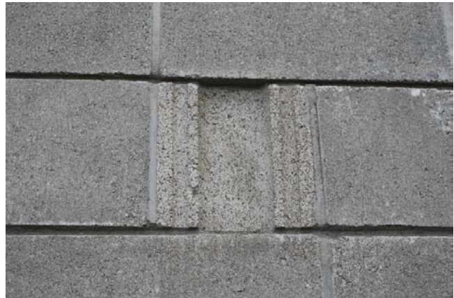
Detail of concrete block
