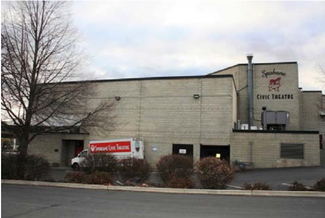
East rear facade, south side, looking west
