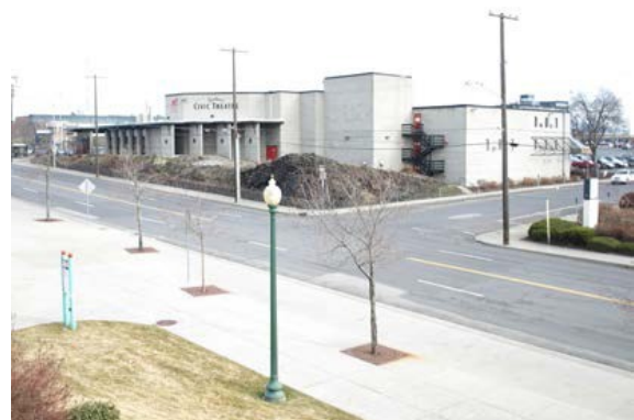
Southwest corner looking northeast
