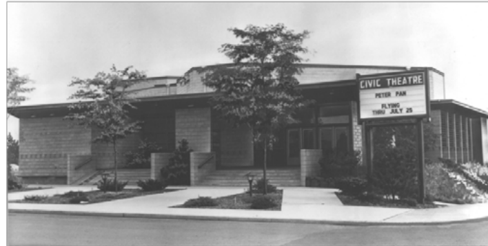
North facade, historic view
