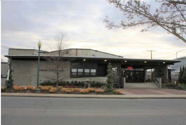
Front (north) facade, looking south
