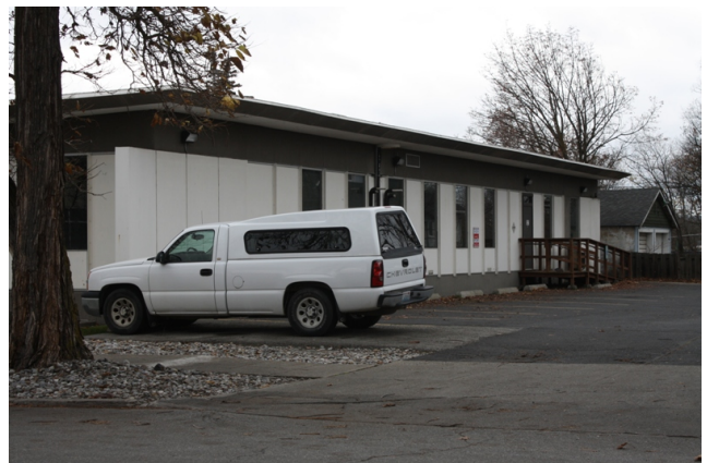
North facade, north wing
