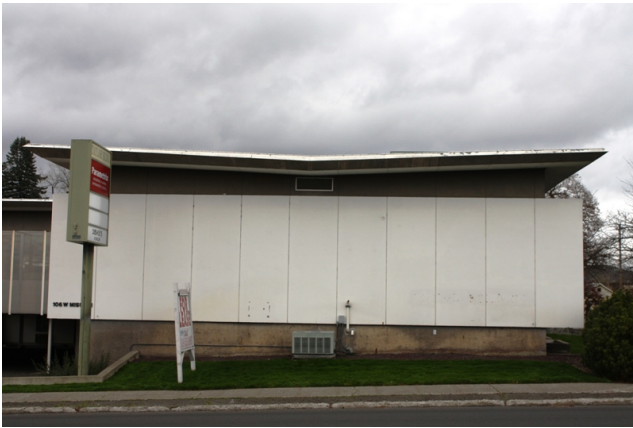
South facade, south wing
