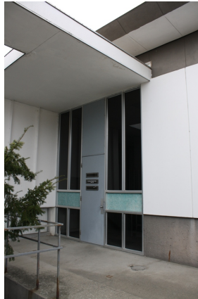
Entry, south facade, north wing
