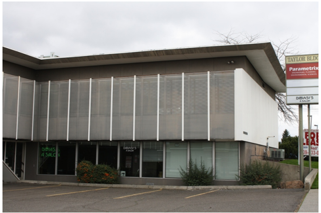
West facade, south wing
