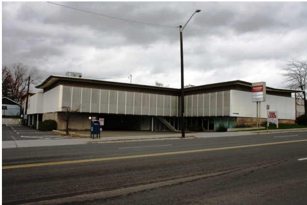
Overview, west & south facades
