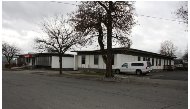
Overview, east & north facades
