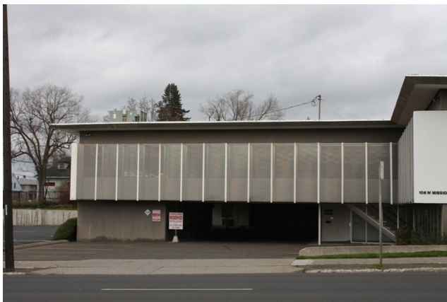
South facade, south wing
