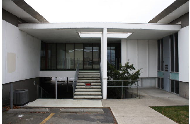
View of bridge entry
