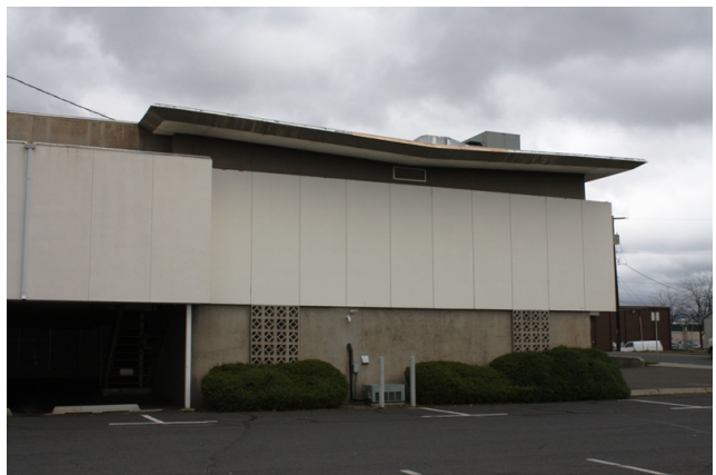
West facade, south wing
