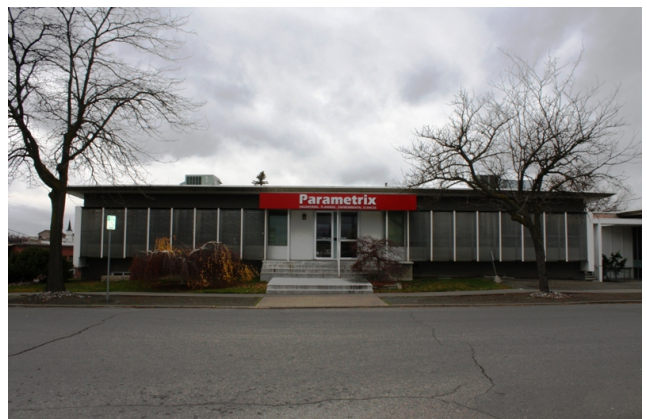
East facade, south wing
