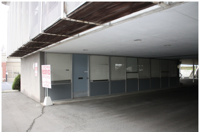
Ground level parking & offices
