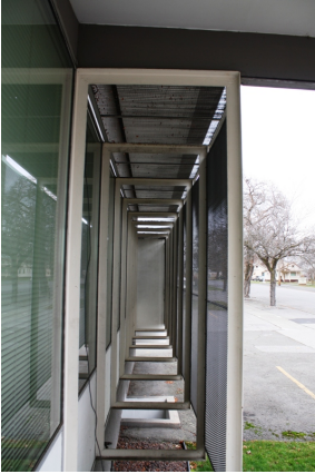
Detail of curtain wall on left, metal mesh screen on right
