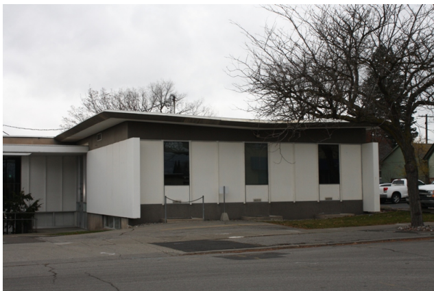
East facade, north wing
