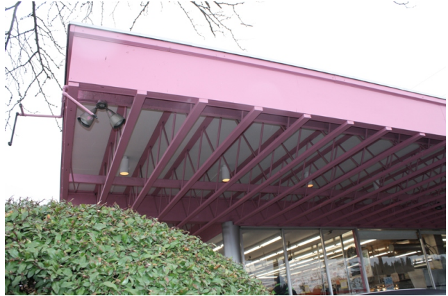
View of space frame roof
