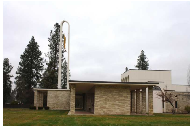
North facade, east end
