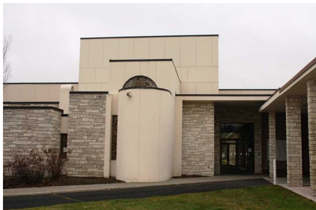
North facade, center
