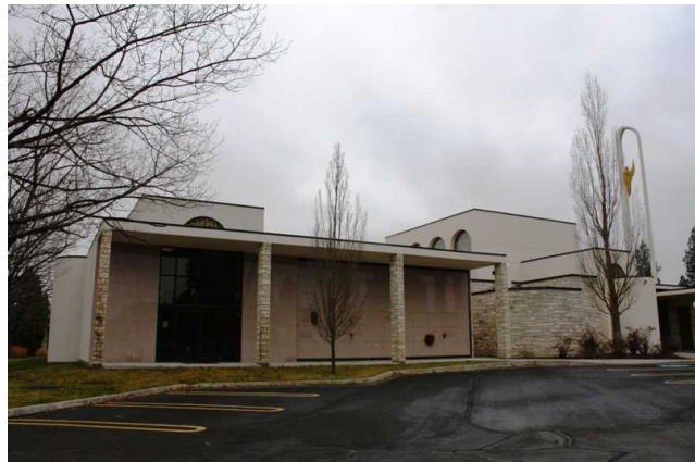
North facade, east end
