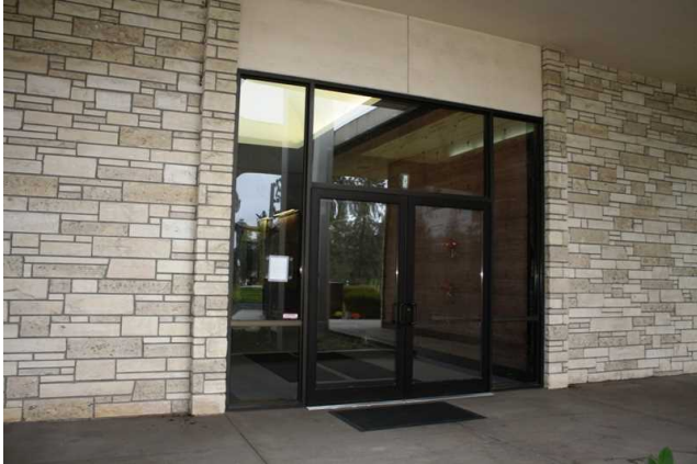
Rear entry, north facade
