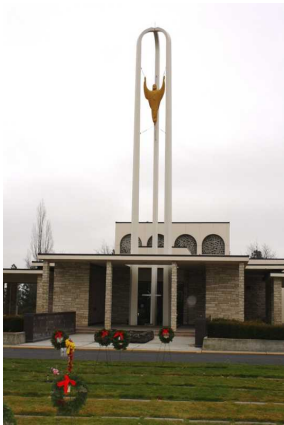
West entry facade
