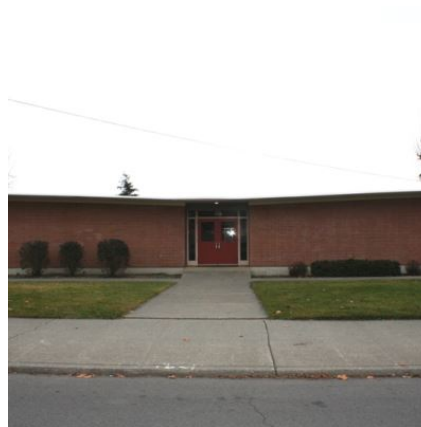
End of classroom wing, typical
