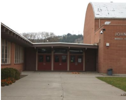
Entry located between gym and south classrooms
