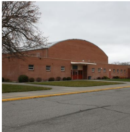
Main entry to gym, looking southeast
