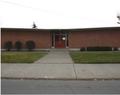
4 - typical entry, west.JPG
