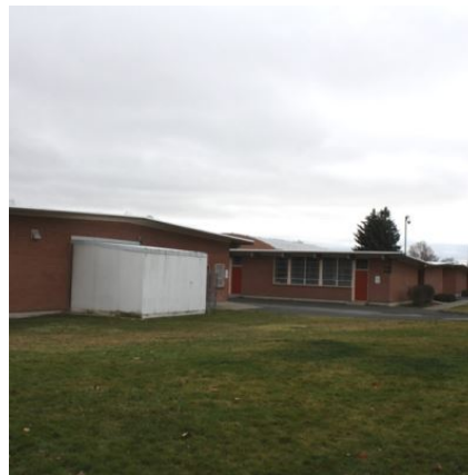
West end of classroom wings
