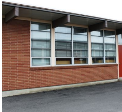
Typical classroom window wall
