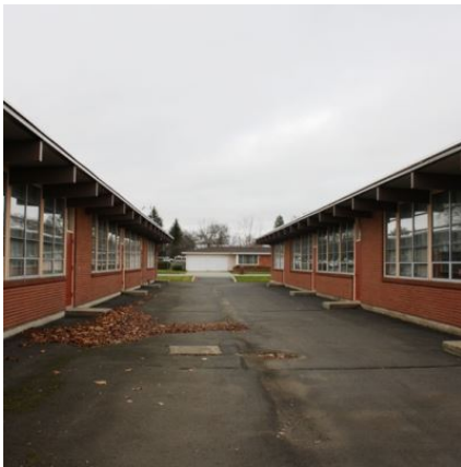
Typical courtyard between classrooms
