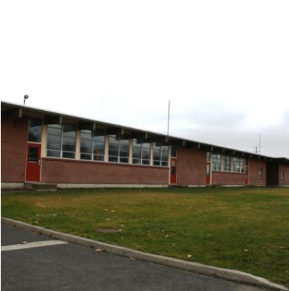
North facade, entry to right side
