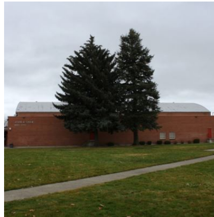
West facade of gym
