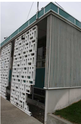
Southeast building corner
