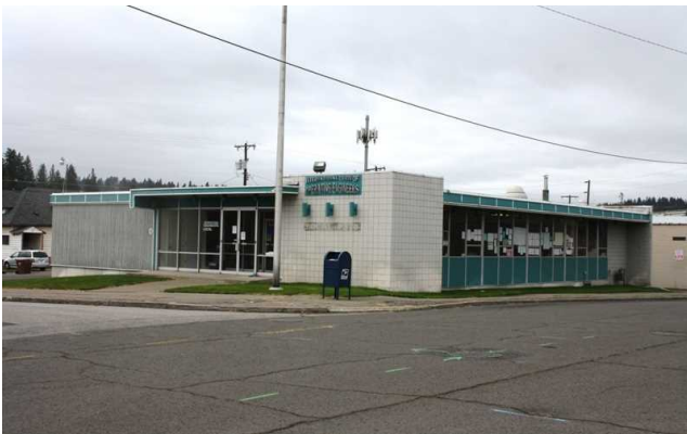
East (front) and north facades
