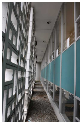
Space between bris d'soliel and rear curtain wall
