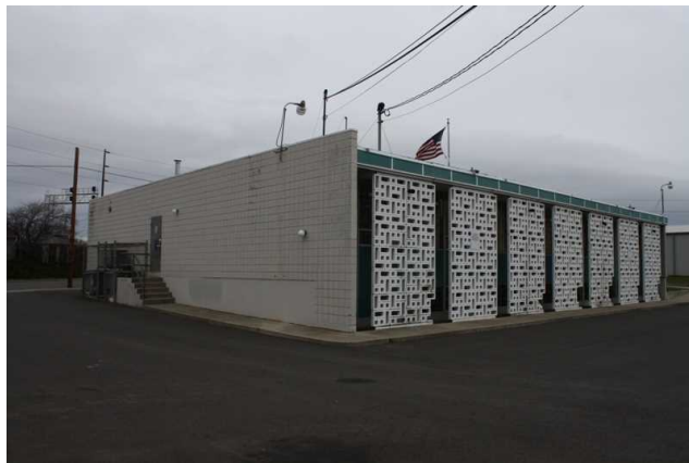
Southwest building corner
