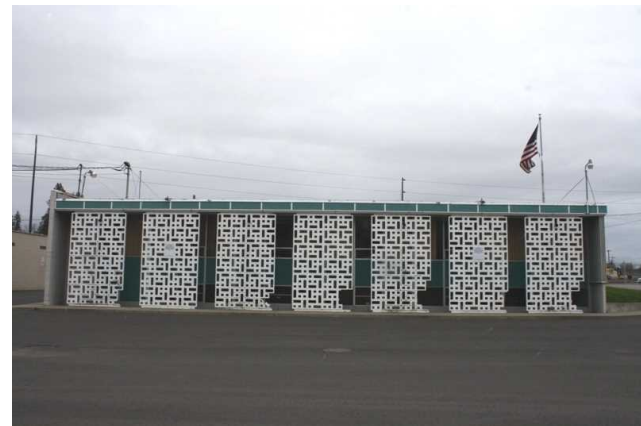
Rear (south) facade
