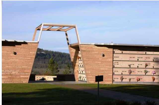
Main building opening, framed view
