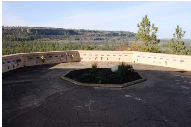
View of octagonal plaza
