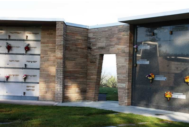
Door opening and view of niches, typical
