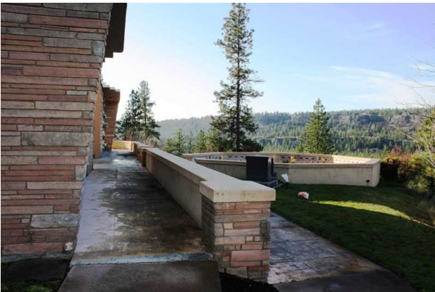
Terraced walkway, east side of mausoleum
