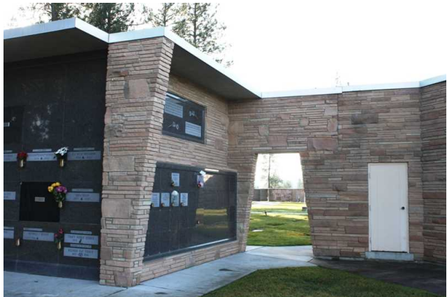
Door opening and view of niches, typical
