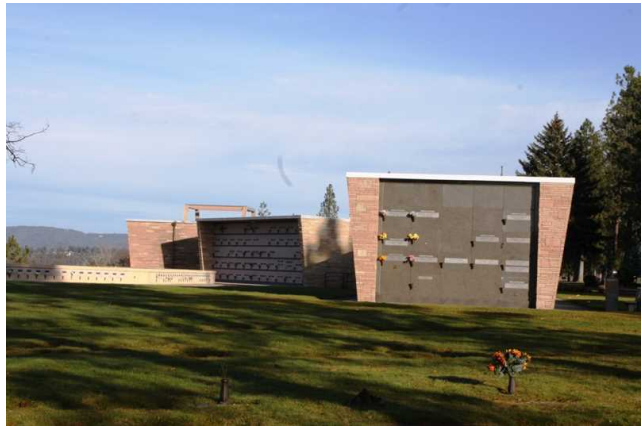
South end of mausoleum
