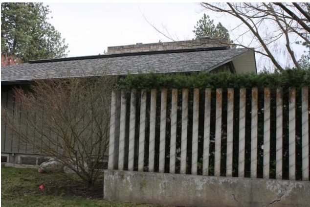
View of chimney detail
