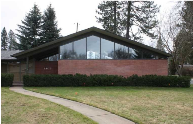
Front facade, west wing
