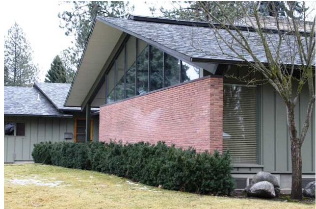
Front facade, west wing
