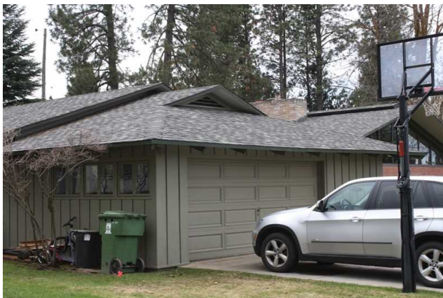
View of garage, east wing
