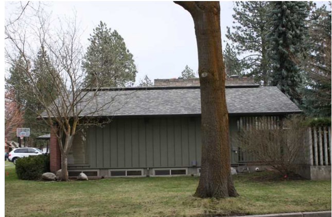
West, side facade
