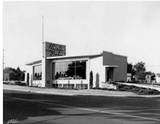
Northwest and northeast facades
