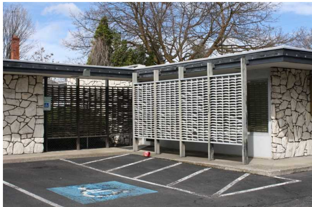
South entry to north building
