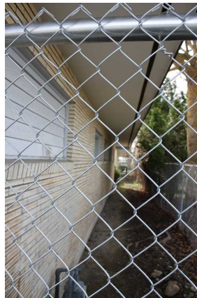
West, rear facade, north building
