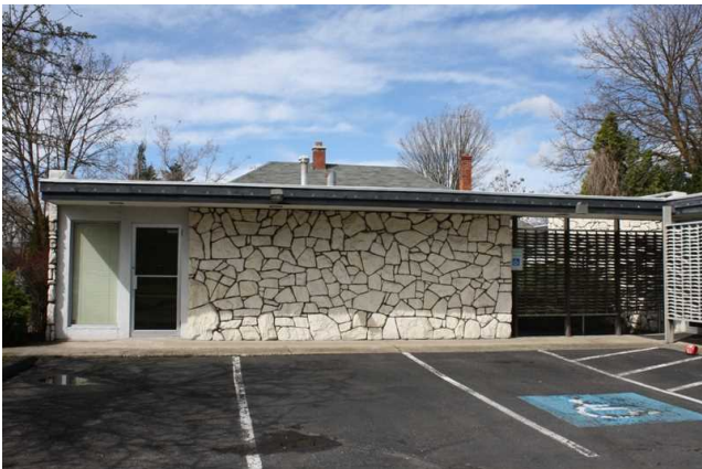
East facade, south building
