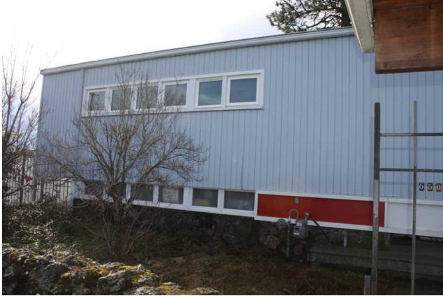
West side of front facade
