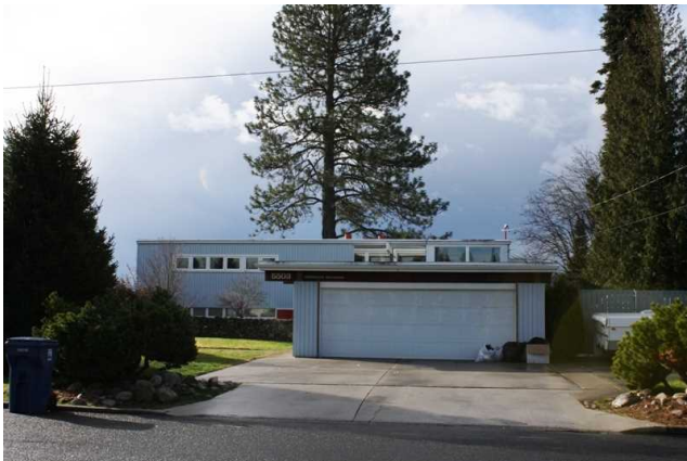
Front (north) facade
