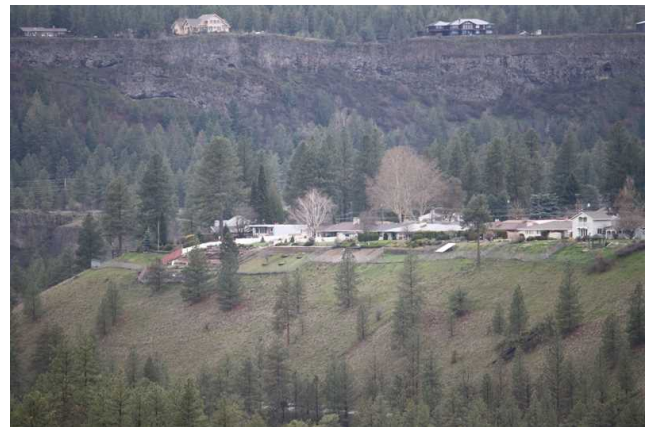
West and rear (south) facades
