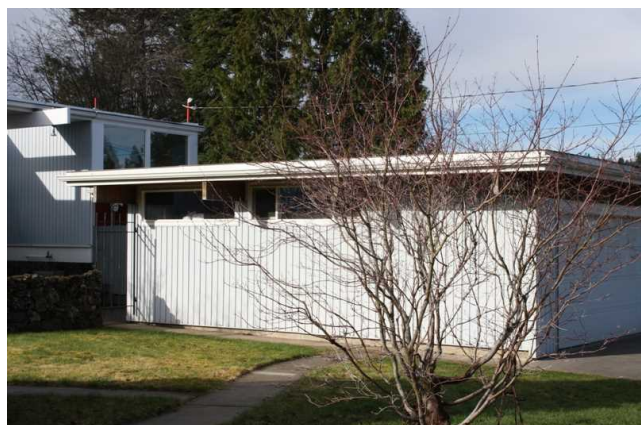
West facade, garage
