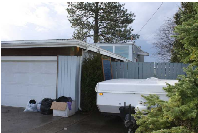
East side facade
