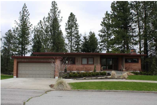
Front (south) facade
