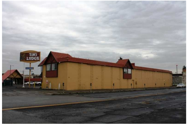
East facade, east wing
