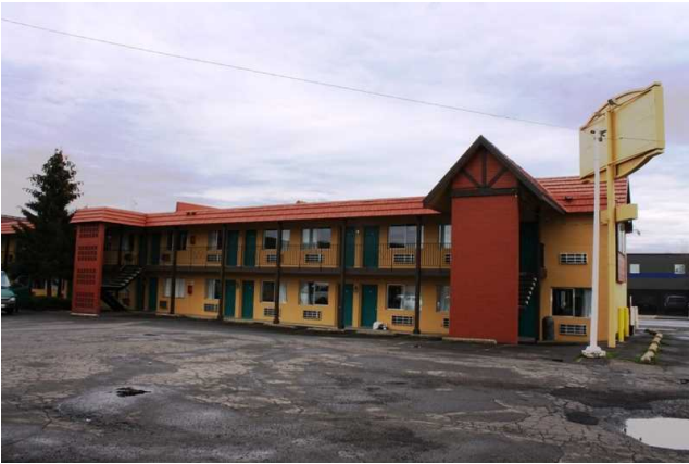
West facade, east wing
