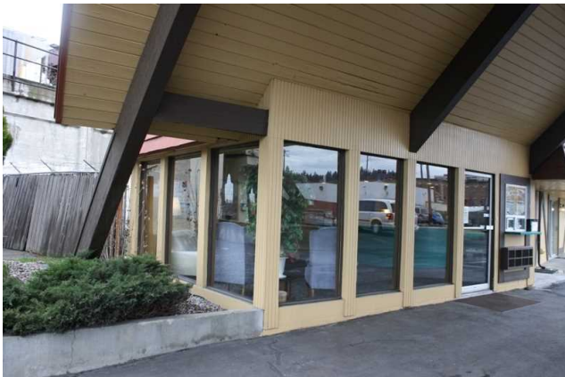
West and south facades, office
