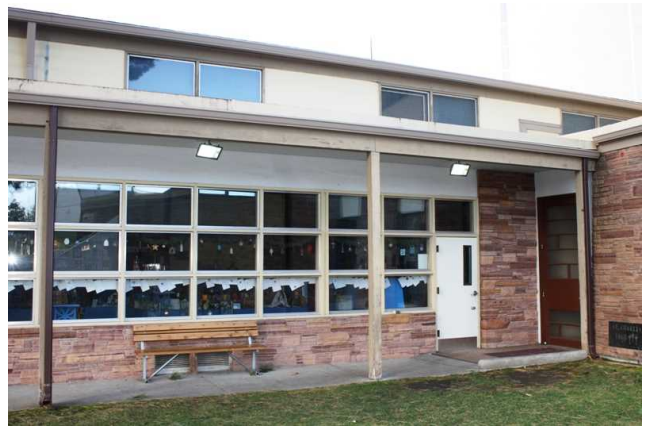
Classrooms south of church
