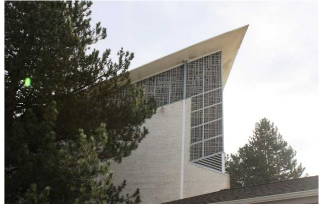
Church, north side facade, roofline
