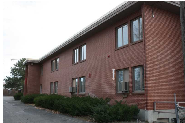
Offices west of church, rear facade
