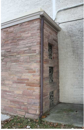
Church, south side facade, detail
