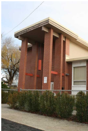
Offices west of church, entry
