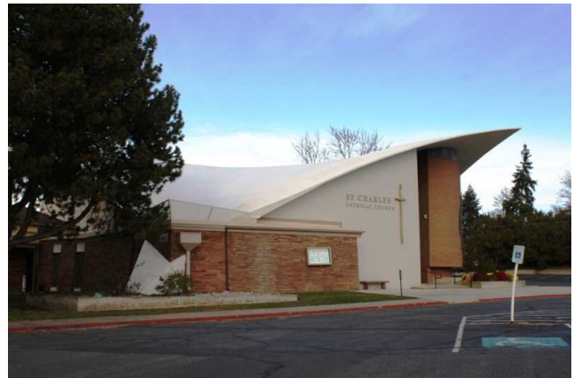
Church, south side facade
