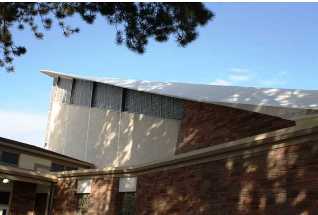
Church, south side facade, roofline
