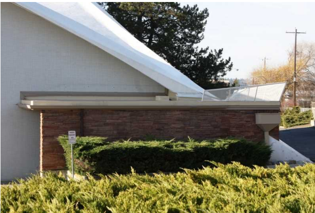
Church, north side facade, detail
