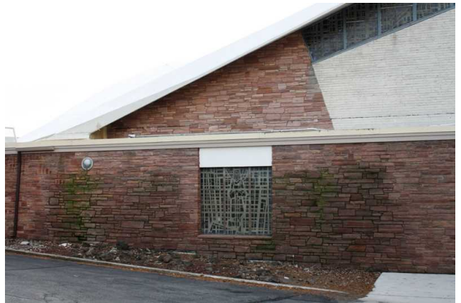
Church, north side facade, detail
