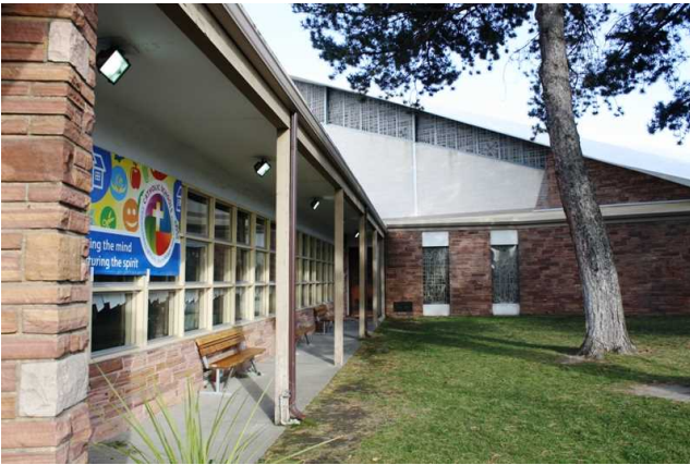
Classrooms south of church
