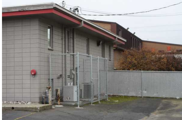
North (rear) facade
