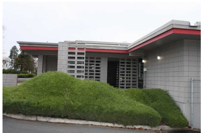
East facade, south end
