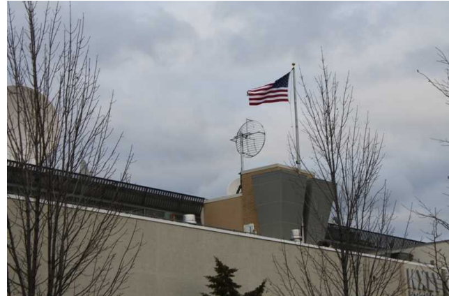
Roof detail, south facade
