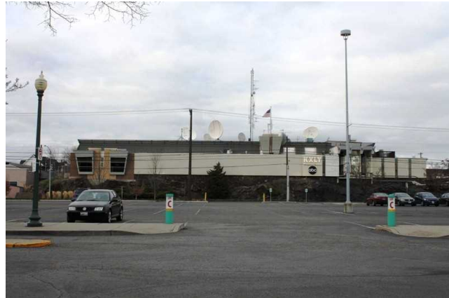
Front (south) facade
