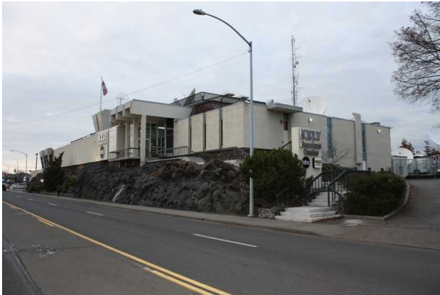
South and east facades
