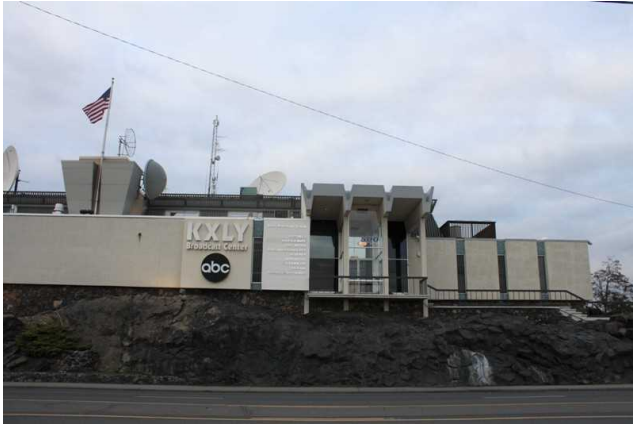
South facade, east end
