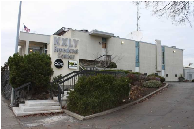
East side facade
