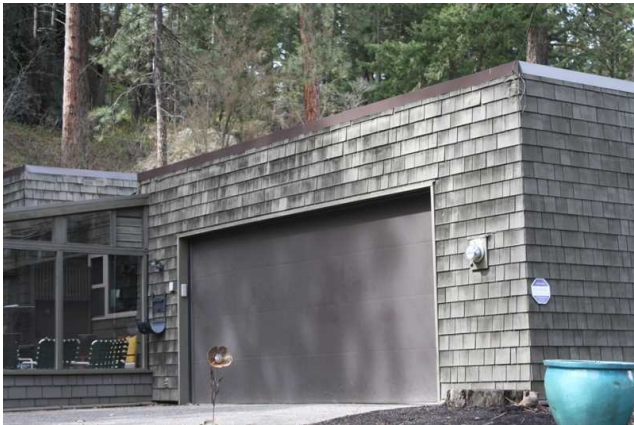
South facade, garage
