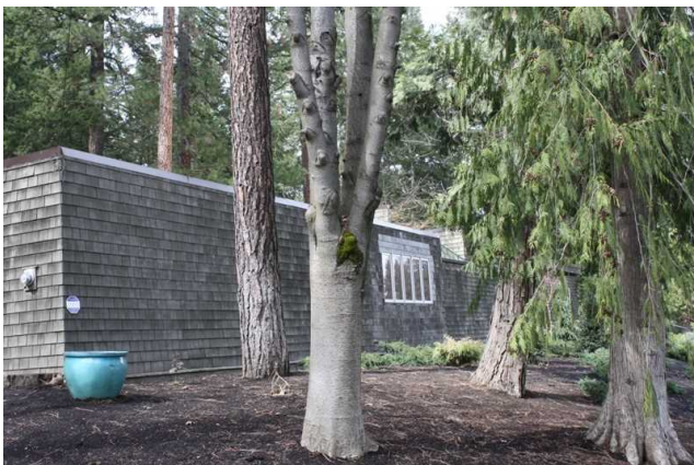
East facade, south end
