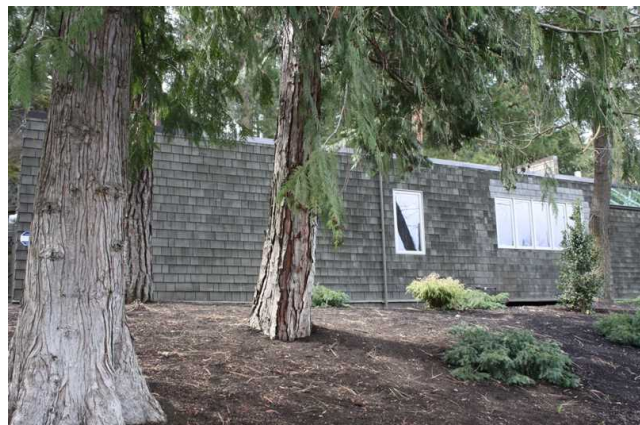
East facade, central portion
