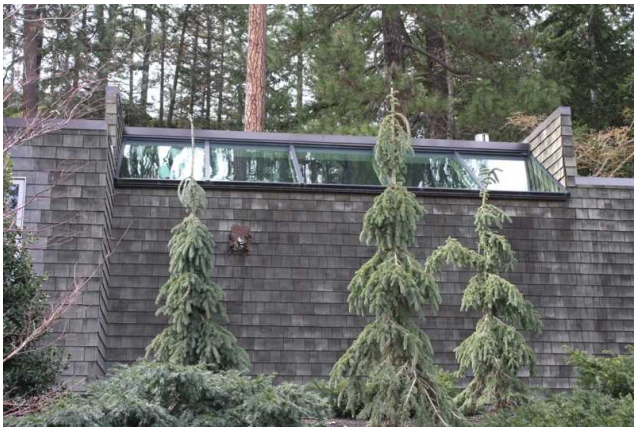
East facade, detail
