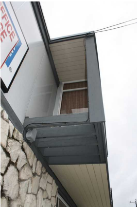
Window detail behind tile panel
