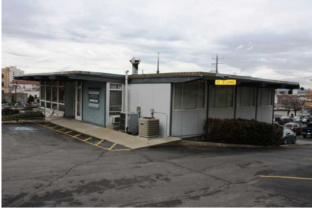
South and east facades
