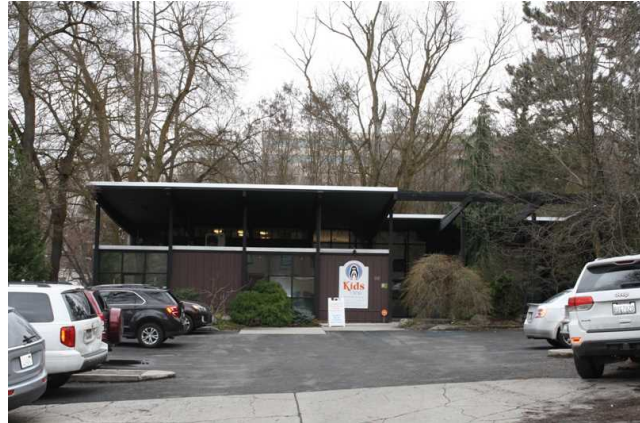
View of west, front facade
