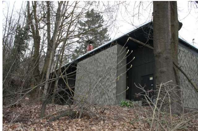
East, rear facade
