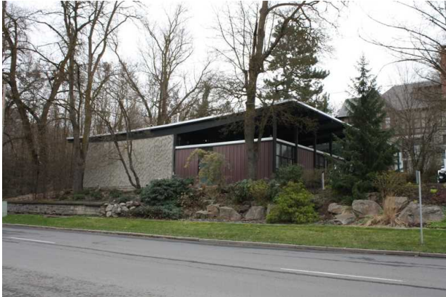
North and west (front) facades
