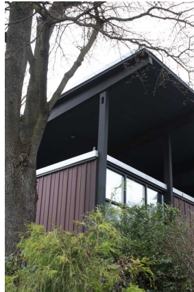
View of addition at northwest corner
