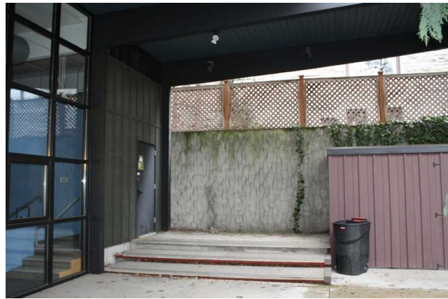
Detail, former stair to Glover Mansion
