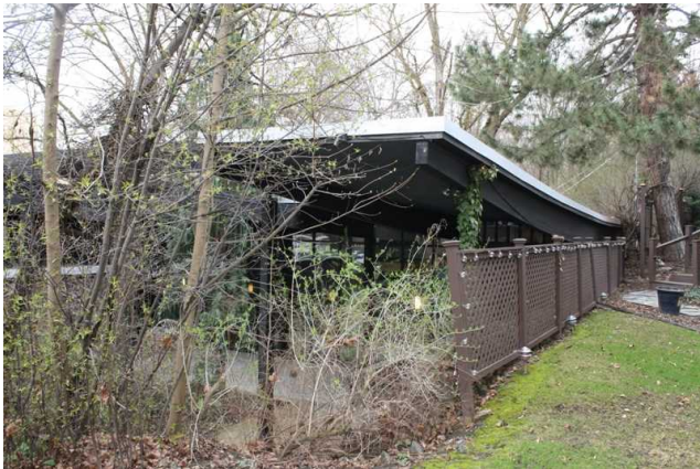
South, side facade
