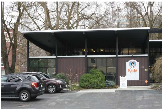
View of west facade, north side
