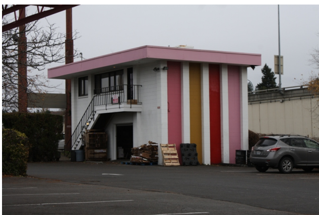
Accessory structure, north & west facades
