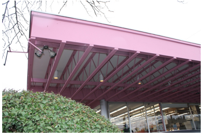
View of space frame roof
