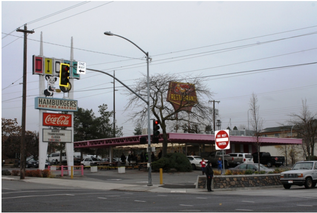
North & west facades
