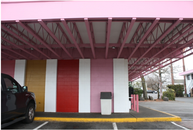
West facade, south end
