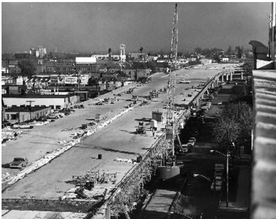
Construction of I-90, Division St exit on right
