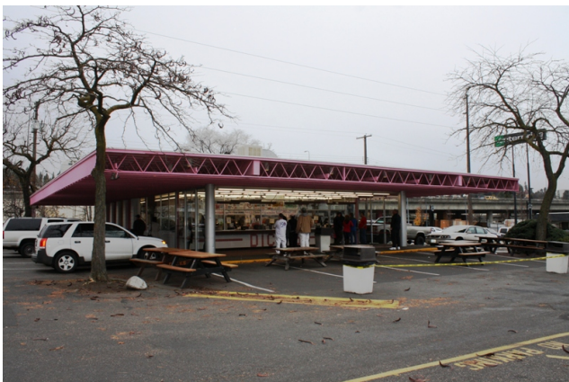
East & north facades
