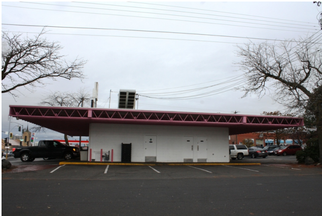
South, rear facade
