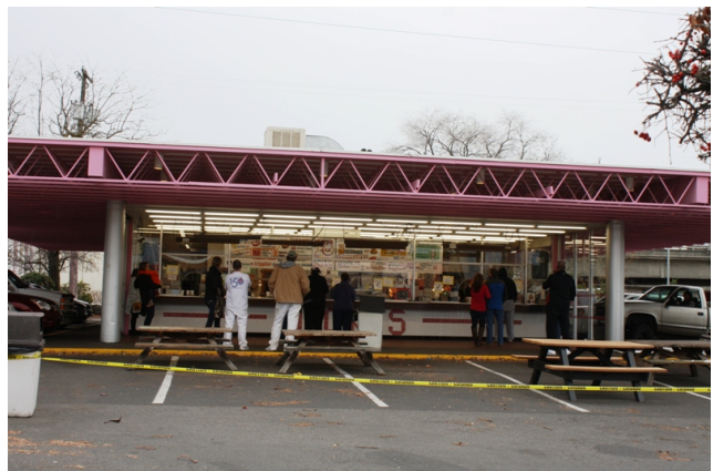
North, front facade
