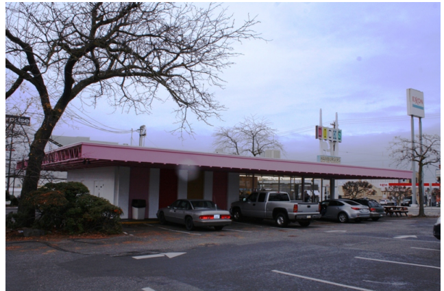
East side facade
